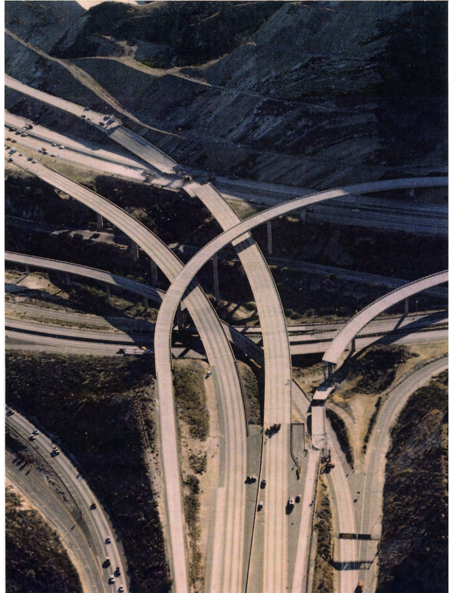
Route 14/Interstate 5 Interchange Collapsed Connectors 53-1964F & 53-1960F
