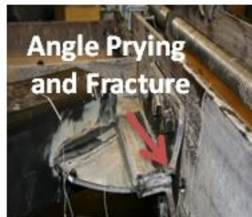
(c) Fracture of Gusset Connecting Angle
