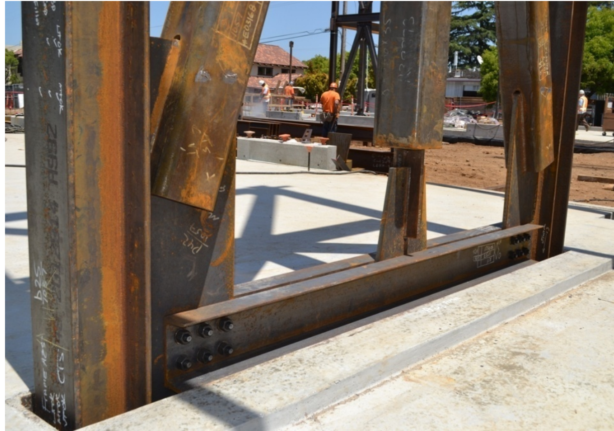
Vertical brace in rocking frame
