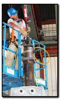
Post-tensioning with threaded bars
