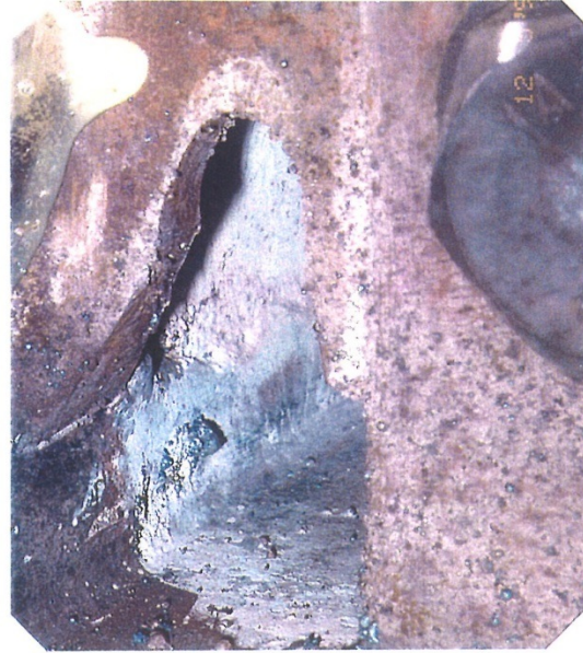
B. Close up of weld access hole and inside weld geometry.
