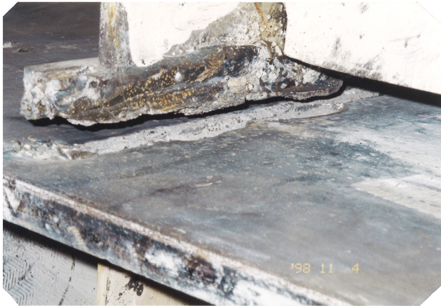
Figure 5. Divot type fracture of connection SP1.1.
