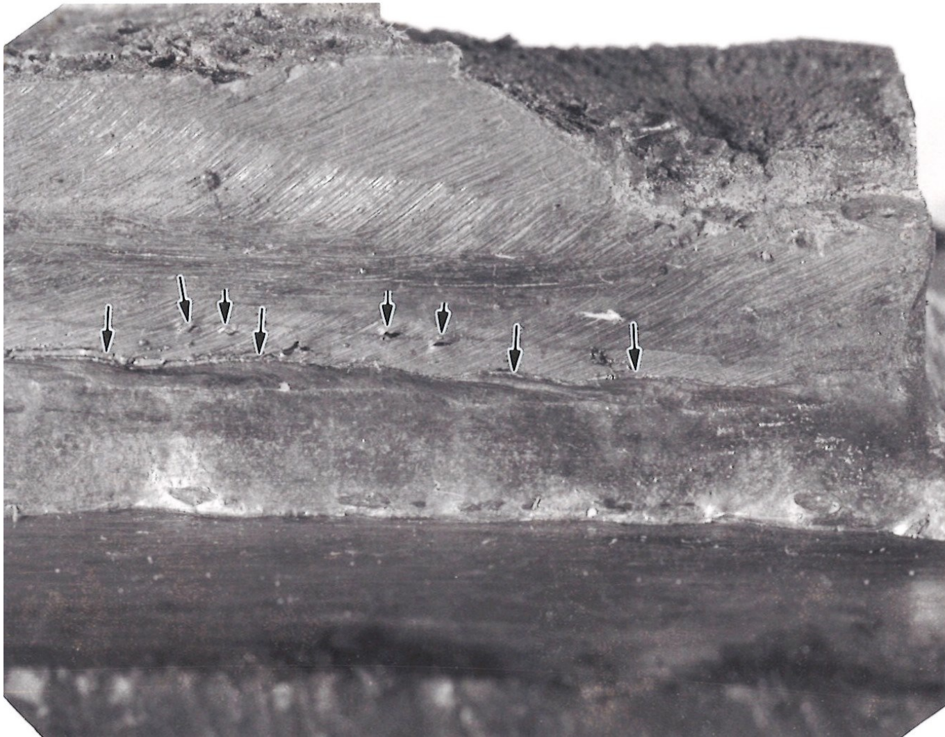
Figure 36. Multiple fatigue cracks along the fillet weld toe and the fusion line of the groove weld.
