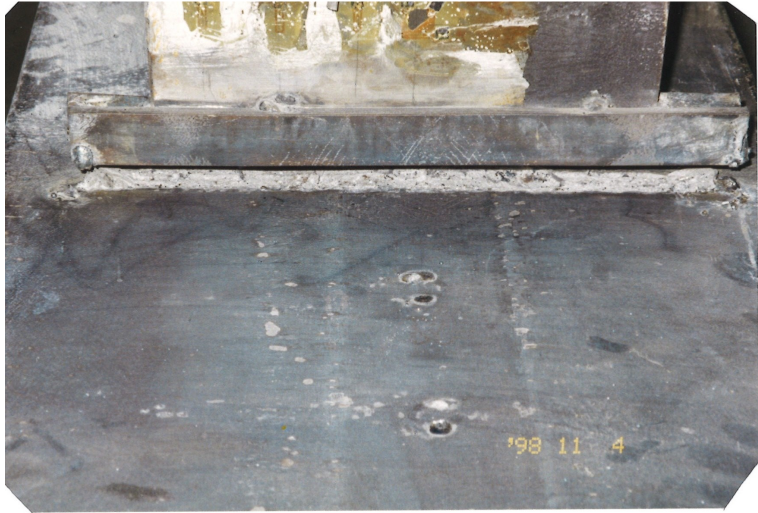
Figure 4. Bottom flange fracture of connection SP1.1 along the length of the backing plate.
