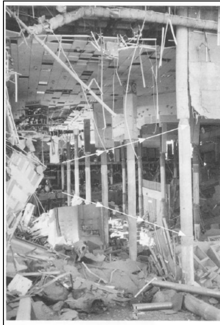
Collapsed interior, Northridge Fashion Center (retail)
