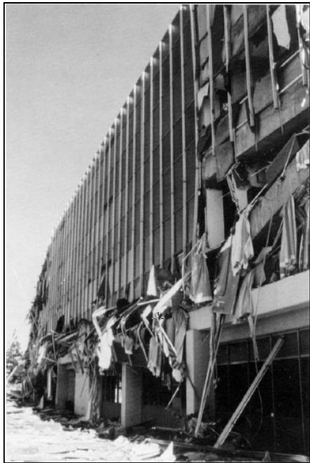
2 nd story collapse, Concrete Frame Building
