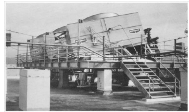
Cooling towers damaged (no occupancy)
