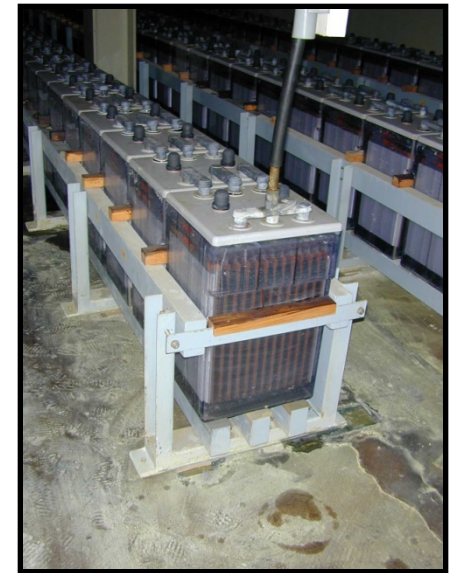
Restrained batteries (Algeria 2004)
