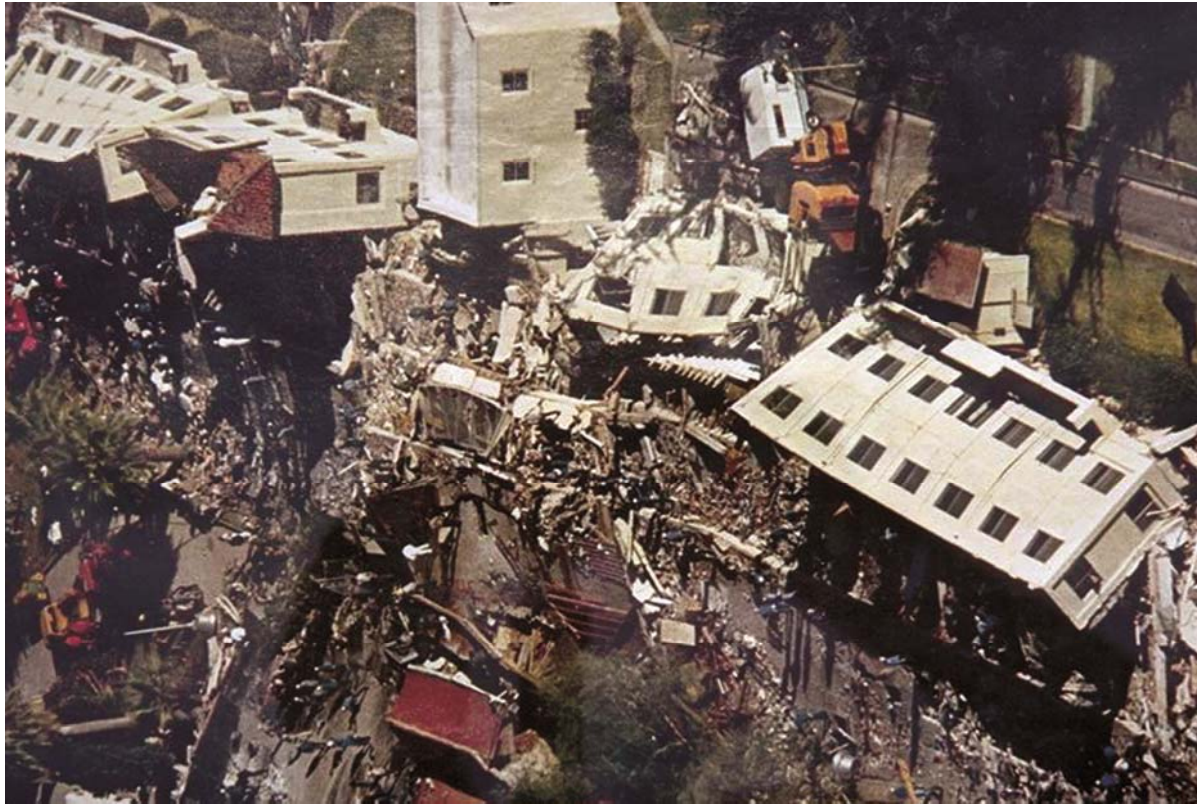
Godden Collection, Earthquake Engineering Research Center, University of California, Berkeley
