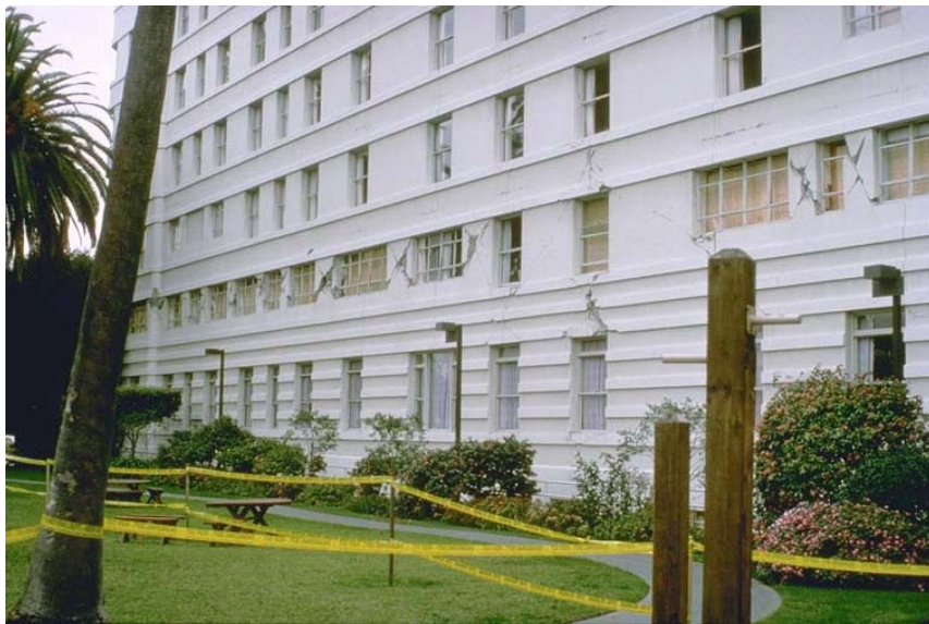
St. John's Hospital damaged in the 1994 Northridge earthquake
