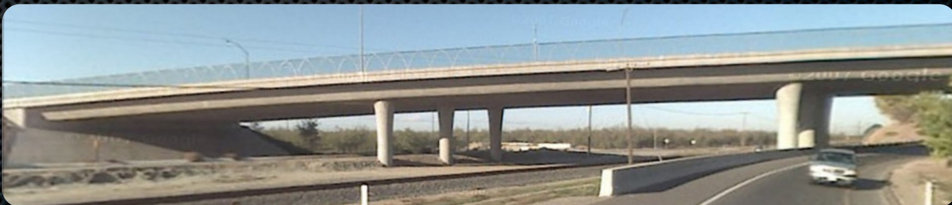
The Jack Tone Road Overhead
